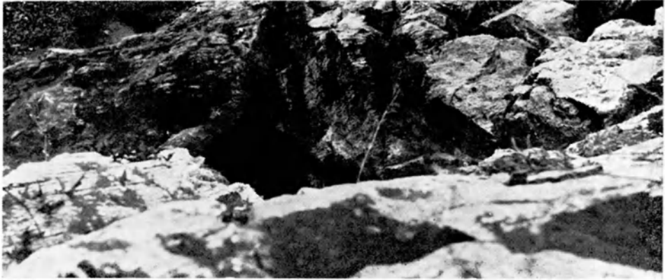
Fig. 21 Bottom of the damaged shaft 7d.
