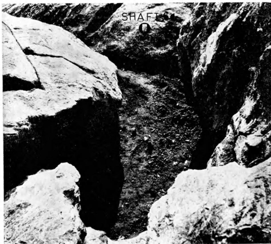
Fig. 20 Access platform of the shaft 6a.
